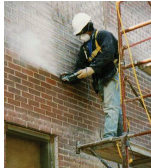
Figure 2 Mason performing "tuck-pointing" on a brick building exterior, using a handheld powered mortar grinder, similar to that used by our patient. Field testing of air levels of dust in similar circumstances indicates that the particle mask shown in the figure may not be adequate to protect against the high levels of dust generated. Photograph courtesy of the National Institute for Occupational Safety and Health.
